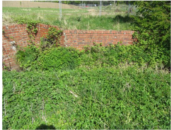
The other side of the Maybury Road culvert
