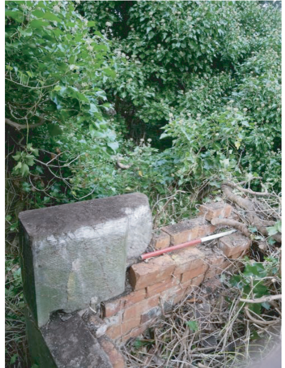
Excavation work within the Walled Garden
