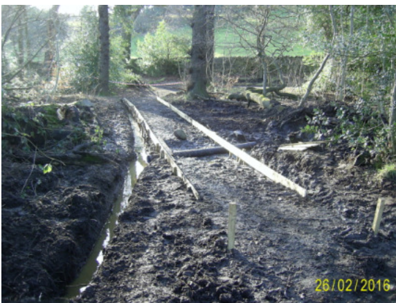
Drainage ditch (left of centre), drain pipe (centre), timber path edging and pathway system at the previous very muddy S.W. corner of the estate.
